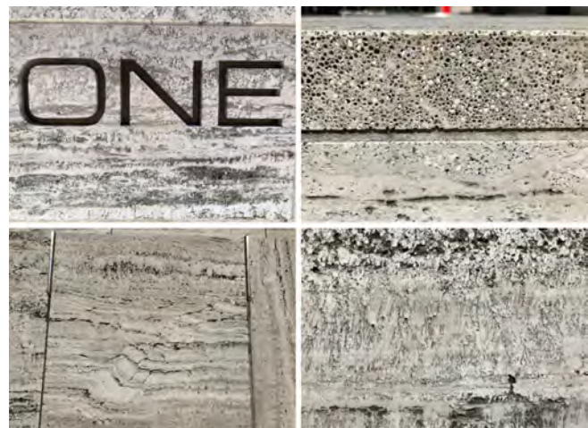
Close-up stromatolite patterns/precipitation growth dominant feature, some vugs partially to fully filled with more transparent cement.
