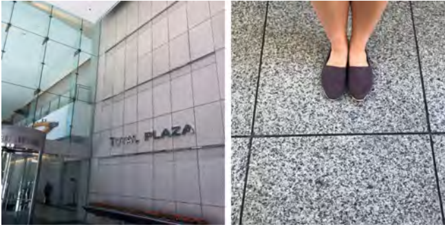
Close-up: uniform medium grained granite containing smoky quartz, plagioclase feldspar, hornblende, pyroxene
